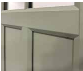
Mechanical mullion to midrail
